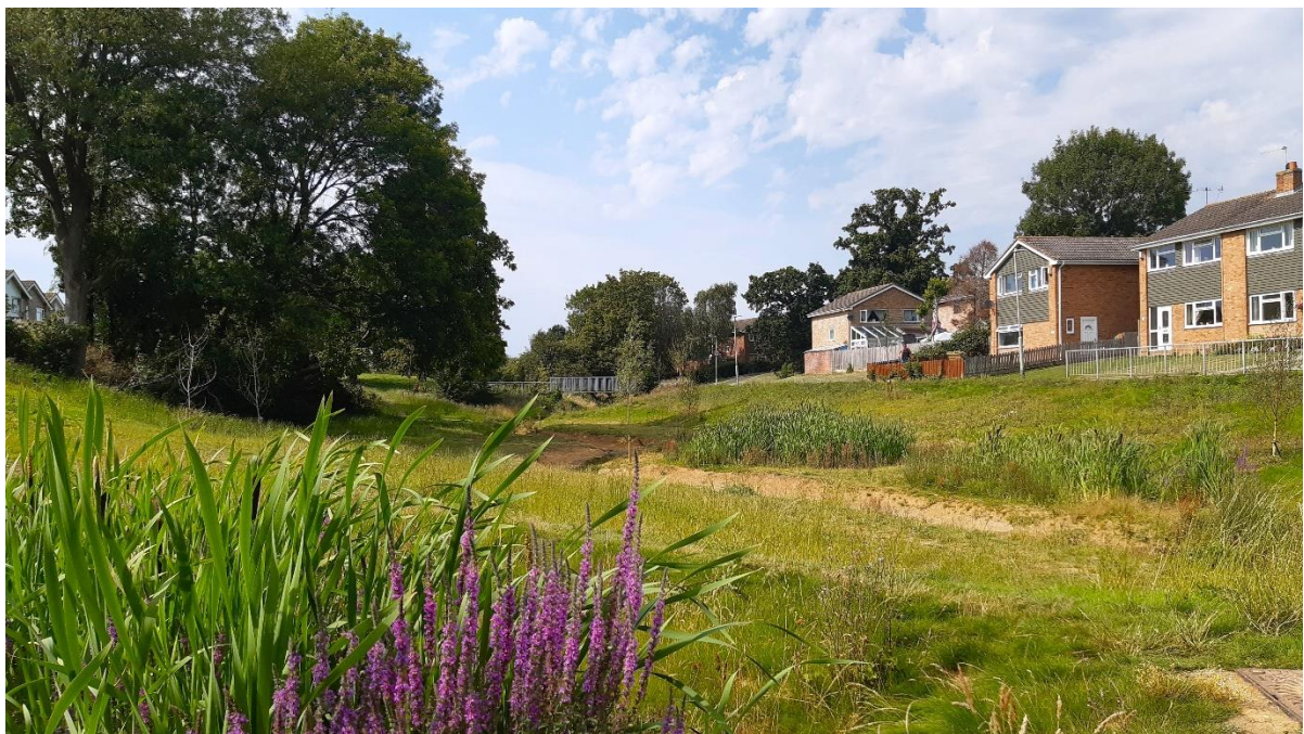
Completed works – natural, sinuous, 2-stage channel, with riparian wildflower meadow
