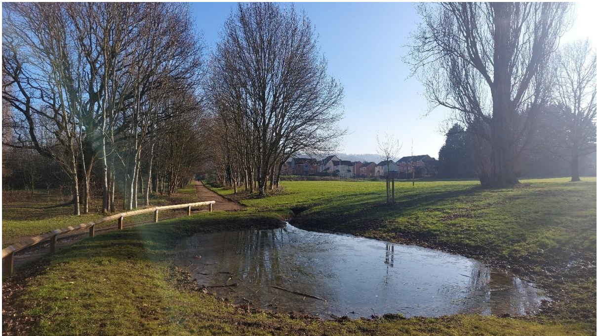
Matson Park SuDS (sustainable urban drainage) Pond
